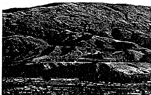
Fig. 7 Landsliding on schist slopes of tectonically elevated Pisa Range at Cromwell (bottom). Pisa Fault (zone) traverses photo below centre, while foreground terraces comprise fluvio-glacial sediments of the last 350 ka. Prominent landslide to left of centre probably is actively creeping. Movement rates of displaced schist indicated by discontinuous transverse ridges are unknown, but on-going creep is likely. Foliation dips towards Cromwell as a result of late Cenozoic folding (photo: G. Randall).
